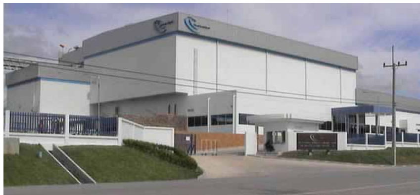
<Photo 2 : MHM's breathable film manufacturing facilities>
